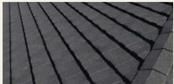
Coloured Stone Tiles Roof
